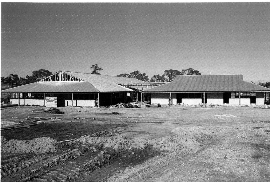
Construction is well underway
