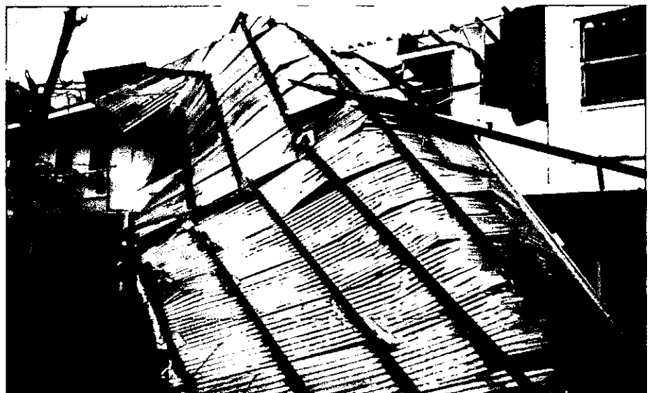
Photo 4: On this block of flats, the leeward roof slope peeled off in one piece, initiated by failure near the ridge.
