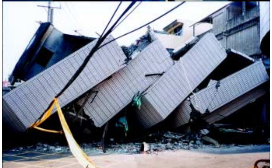
While traveling through the streets, the teams observed the random collapse of structures. Perhaps one or two buildings in a street had suffered major structural damage whilst the others were relatively intact.
