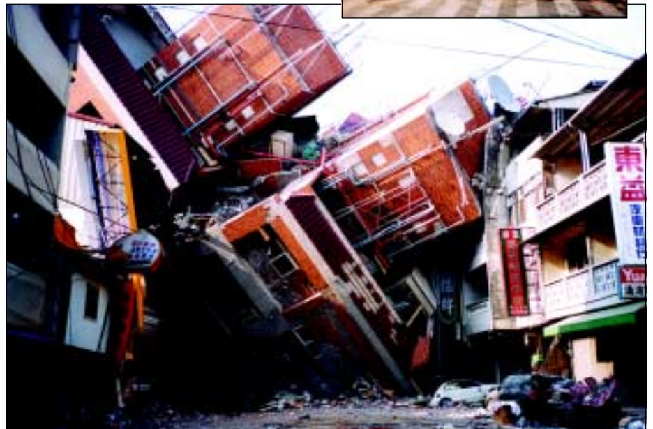
Above, inset: The quake of September 21, and subsequent aftershocks, caused the destruction of 10,984 structures and the partial collapse of 7563 buildings.
