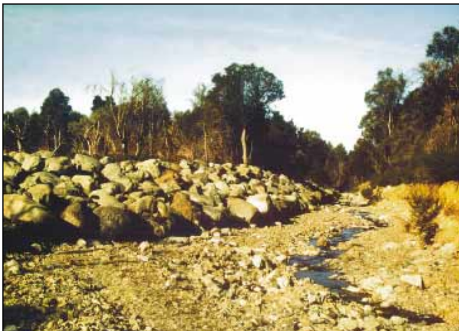
Figure 2(a): Kowhai Stream in 1985 showing the recently completed protective works.
