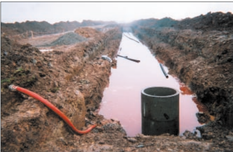
Figures 6 & 7: mass graves were used, but in at least two instances, in Durham and in Wales, it was reported that the bodies would have to be dug up again because of the risk of pollution of the water table.
