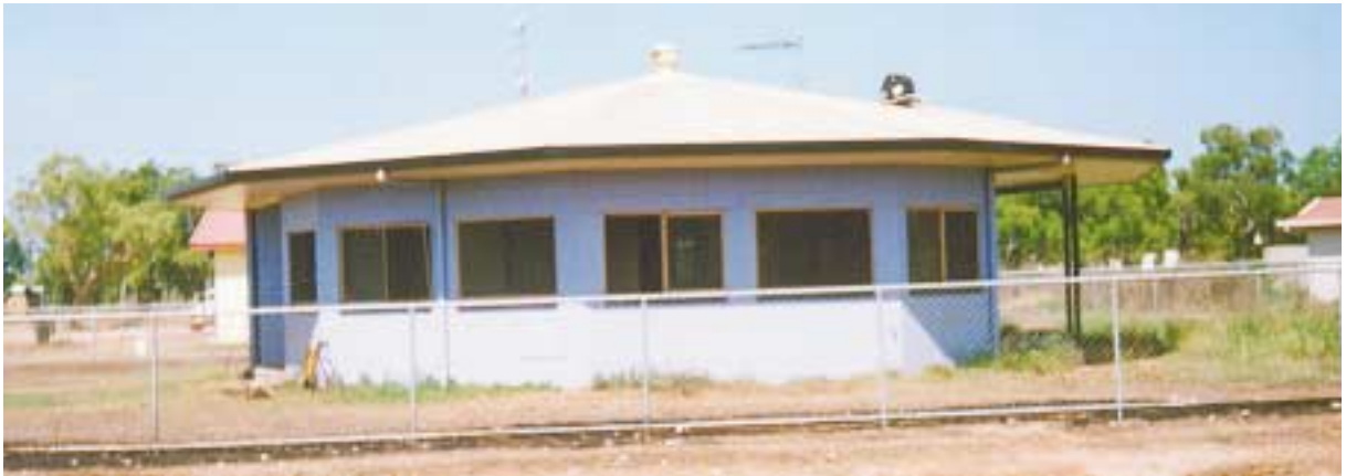
House built post-cyclone Ted (1976).
