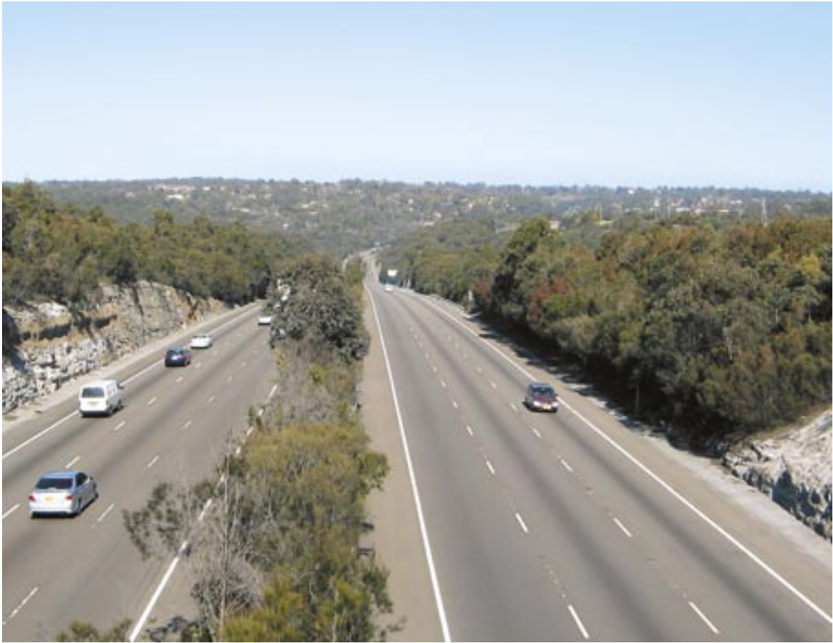
The Sydney – Newcastle Freeway (F3) is often closed due to severe smoke and bushland fires surrounding the road during peak seasons. As this is the only main roadway linking Sydney to Newcastle, extensive delays occur.
