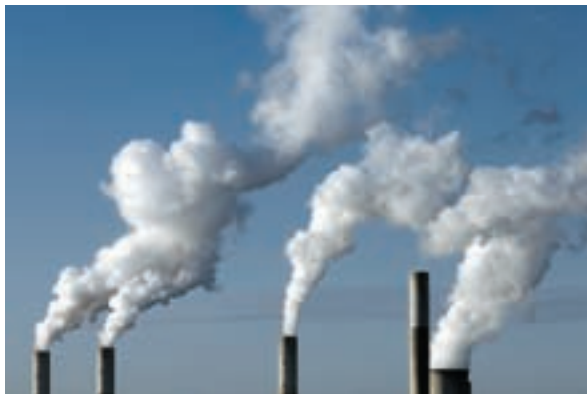
Hazardous airbourne pollutants.
