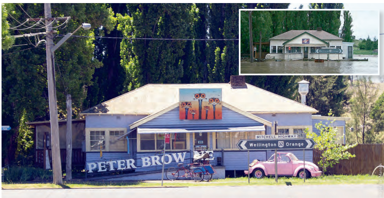
Flood waters reached the front door sill of the gallery at the intersection of Gidley Street and Mitchell Highway.
