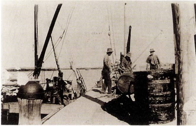
Unloading beer from a lighter at Cossack's jetty. The cargo ketch 'Battler' about to depart from Cossack. The lighter 'Nicol Bay' which brought cargo from ships anchored about eight kilometres away. The abandoned Customs House.
