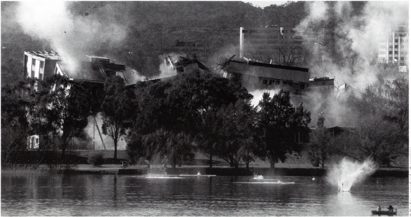
Canberra Hospital Implosion
