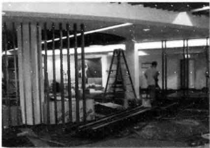
Construction at Curtin
